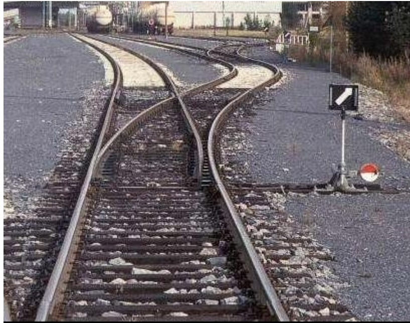
Figure 1. A switch is moved to cause a conventional train to change tracks. Picture of switch is from Wikipedia®
